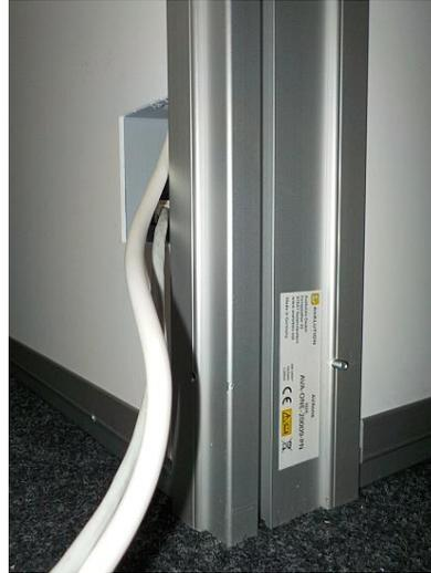
Place the 45x45 profile like in the picture, so that the screw is facing towards the inside of the cabin.
