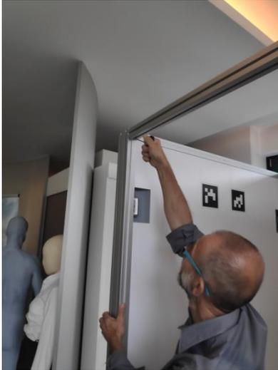
Place the ladder on the front side and mount the third 45x45 profile in the same way as before.
