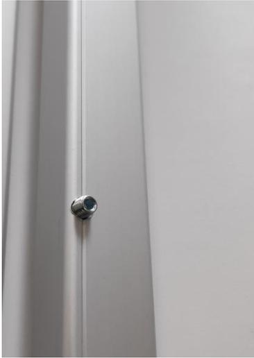
Tap the profile slightly with a rubber hammer to fit into the groove.
